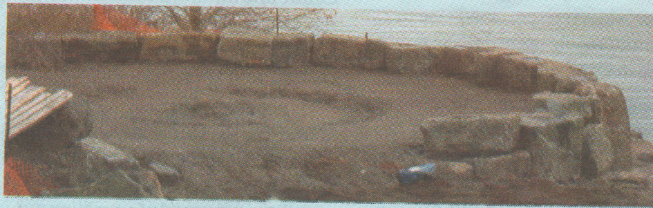
Work is well underway on the ceremonial fire pit.
